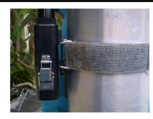
View 2 shows the 2010 Comms Bracket with the comms box mounted (side view).
